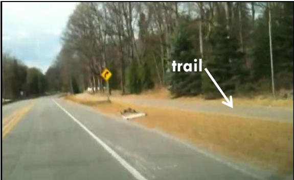
A separated trail might look something like this section of the Little Traverse Wheelway along M-119 between Petoskey and Harbor Springs
